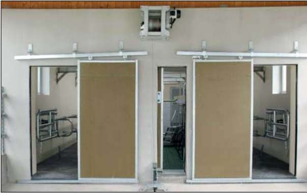
▲ Wall fastening drive winch EW4
