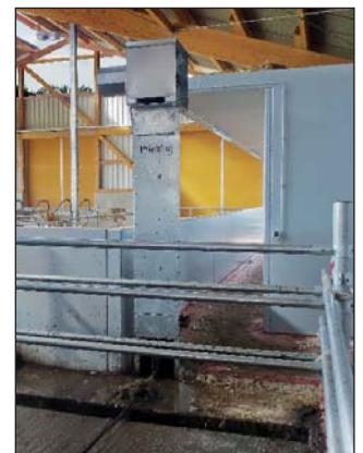
▲ Drive winch EW4 on floor console
