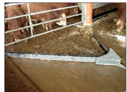
▲ V-scraper on the walkway
